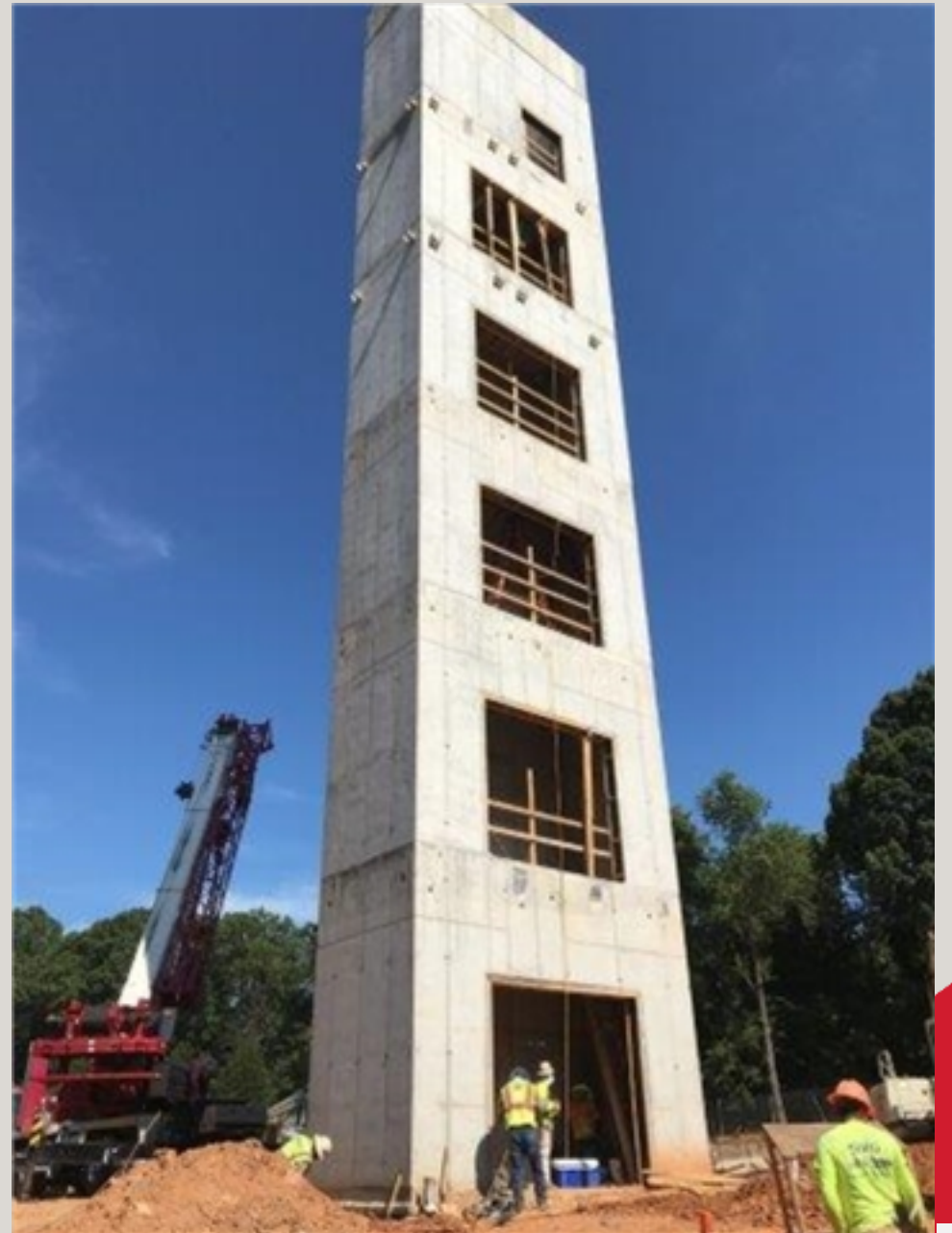
Elevator Hoistway Forming Complete
