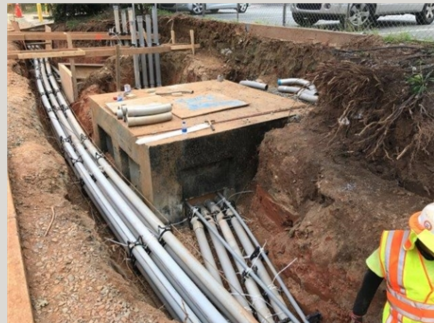
Installing Electrical Ductbank on Cromartie St.
