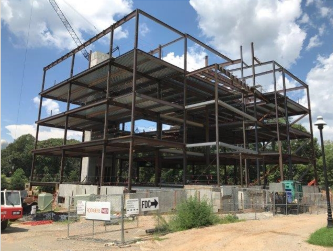
Erecting Steel Super Structure
