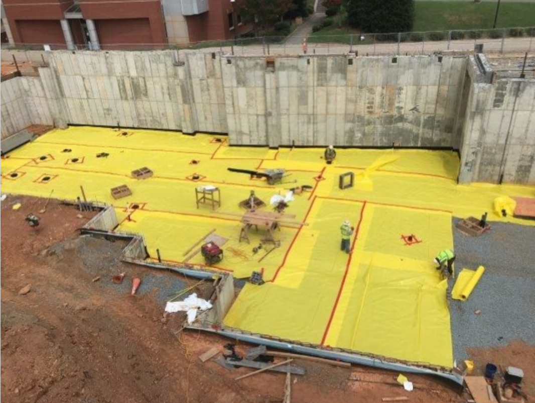
Installation of Waterproofing at Basement Level
